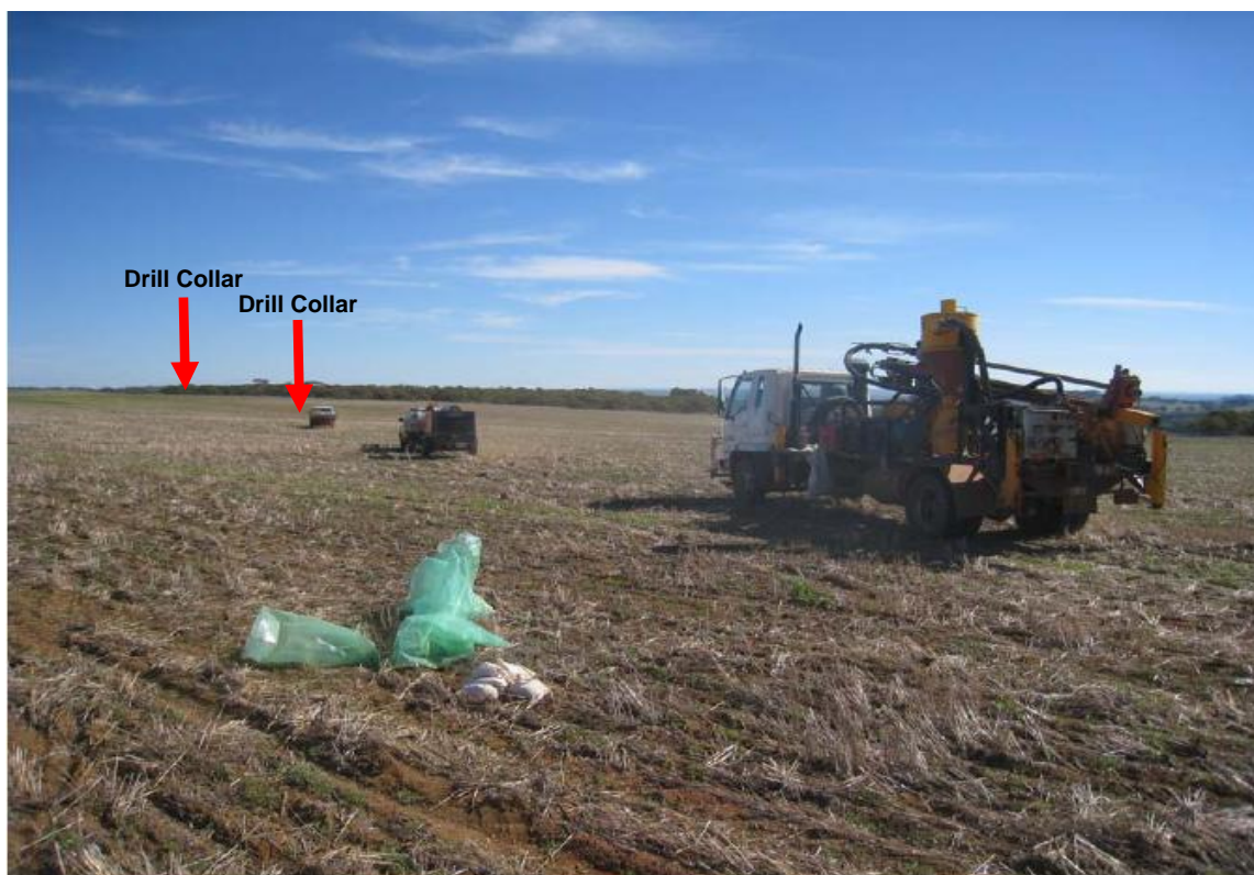
Figure 4 – Mobilised AC drill rig highlighting very low ground disturbance and 200m collar spacing.
