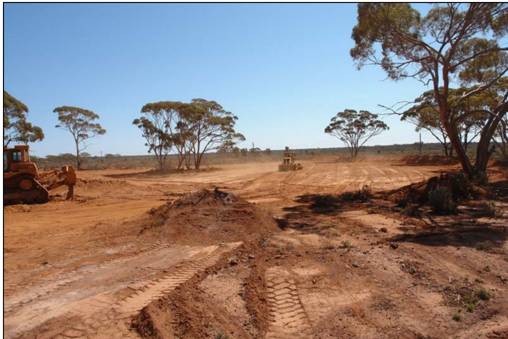
Figure 2: Surface clearing at Costello Open Pit.
