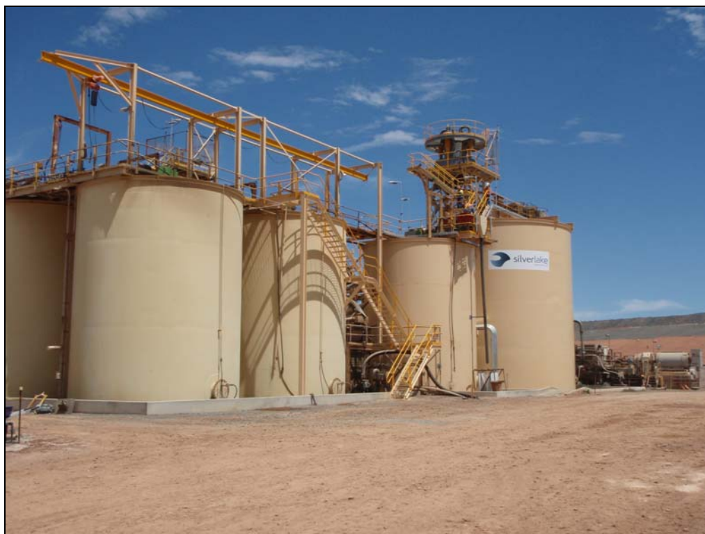
600,000 tpa Lakewood Gold Processing Facility
