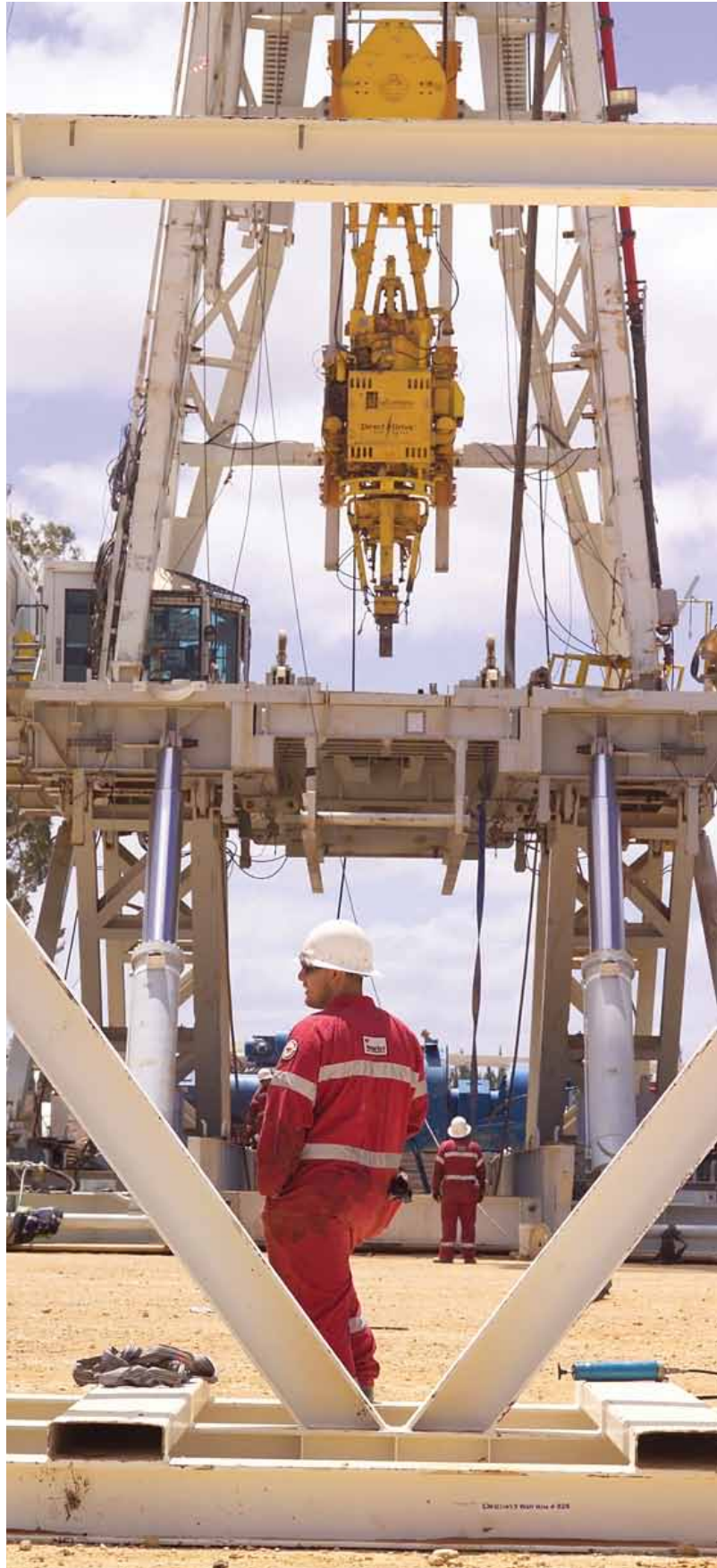
Contract drilling rig (Weatherford) Salamander-1.
