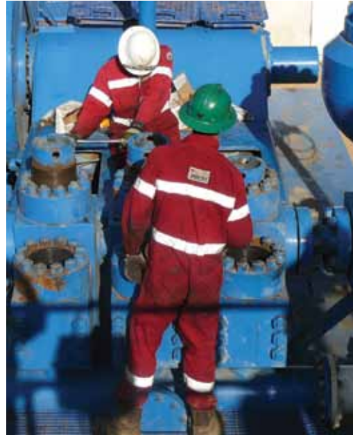
Installing mud pumps.
