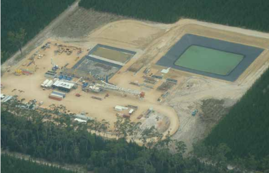
Salamander-1 well site, with rig mast (55m) still on the ground. The large lined pond (14MI) is constructed for the well testing programme.
