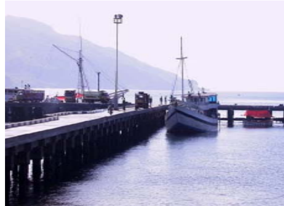
Port facility Ende, Flores
