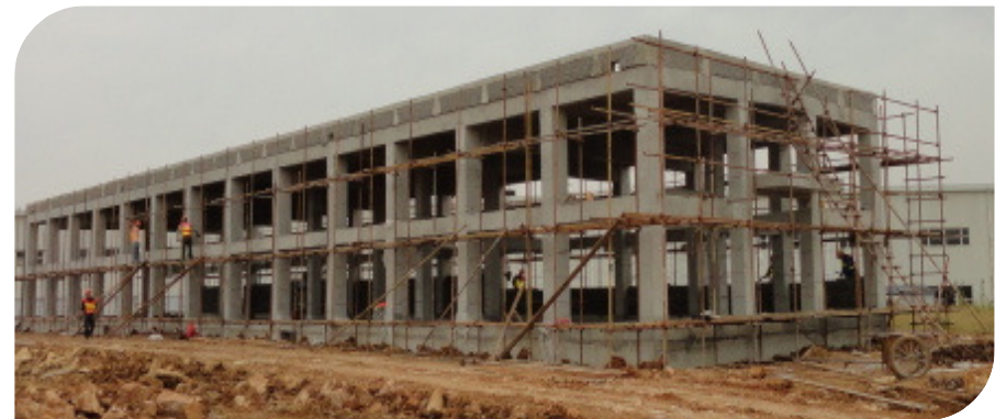
Xuzhou Foundry Under Construction
