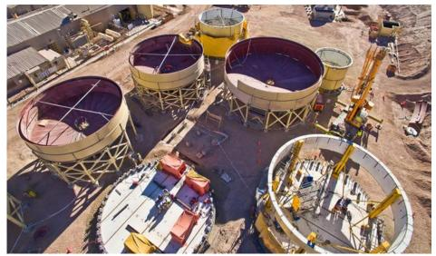
Figure 3: View of the agitation leach plant being constructed at Guanaco mine site
