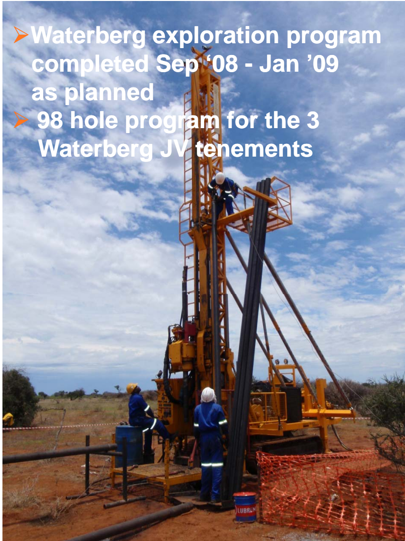
Core Drilling on Waterberg No.1
