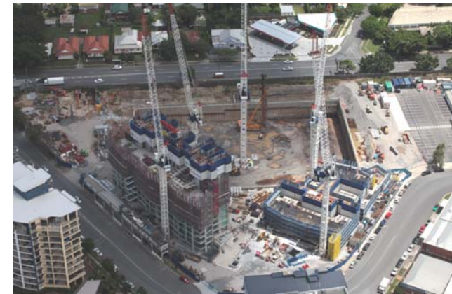
Hamilton Harbour Construction – Brisbane, Queensland
